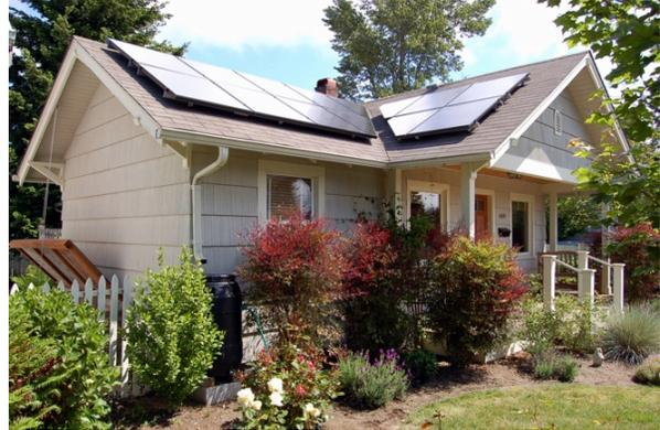
*Installing solar panels to face the west in addition to the south can reduce pressure on grid and enable solar power to satisfy a portion of peak afternoon demand. Image credit: NREL/Brothers Electric © 2008*
