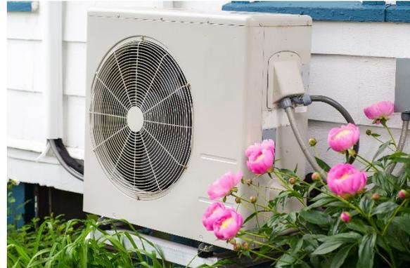
Figure 4. Residential air-source heat pumps transfer heat between the outside air and the home.
